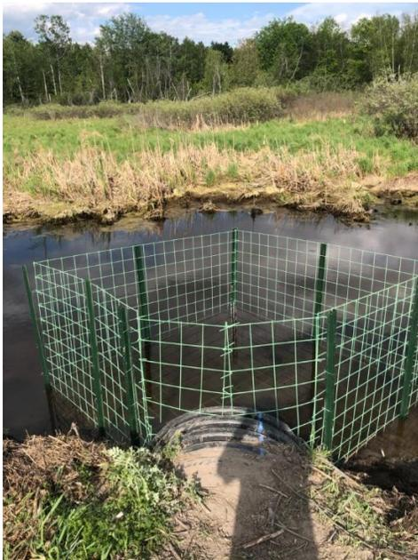
This diamond shape enclosure is meant to “deceive” beaver and discourage the building of a dam.
